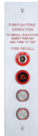
Intermediate hall station with fire services devices
